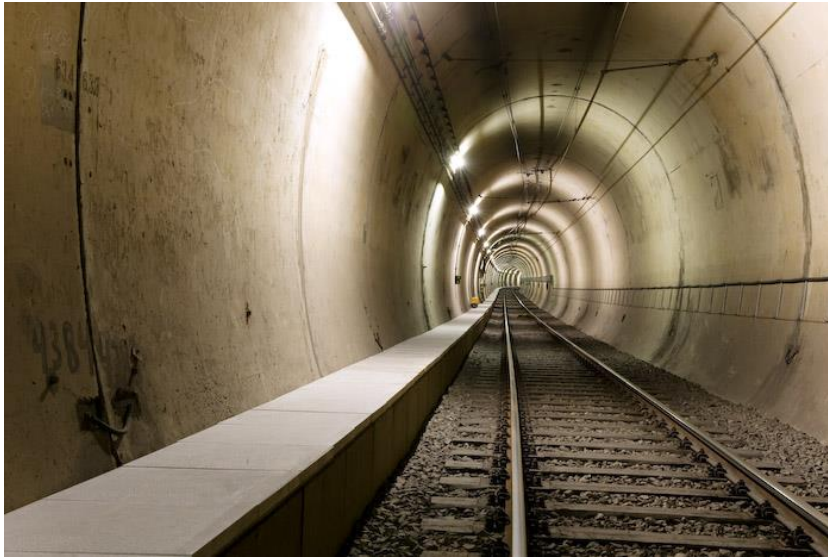
Bored Tunnel Example
